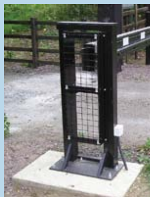
Above: Barricade Beam Cabinet foundation
