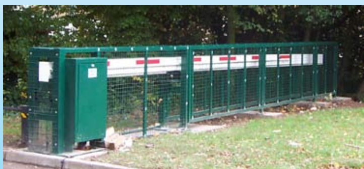
Runback of Barricade Beam fully encased in pedestrian guard rail to ensure no trapping areas.
