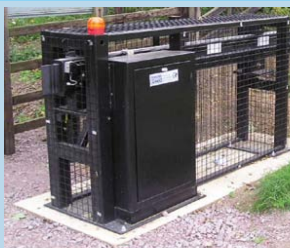
Above: Barricade Beam Cabinet foundation
