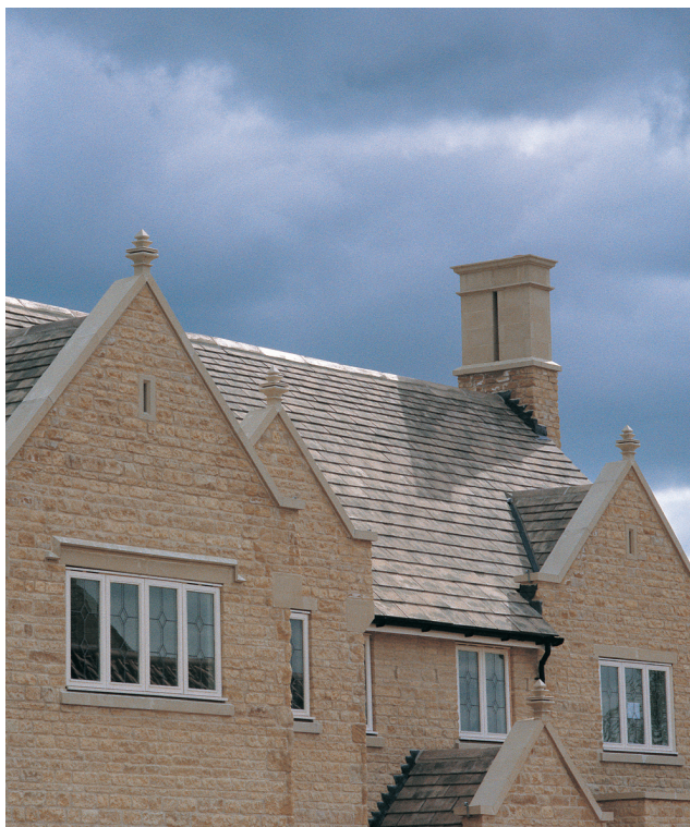
Hardrow® Slates Duets™ Barley laid on Bastion Homes
