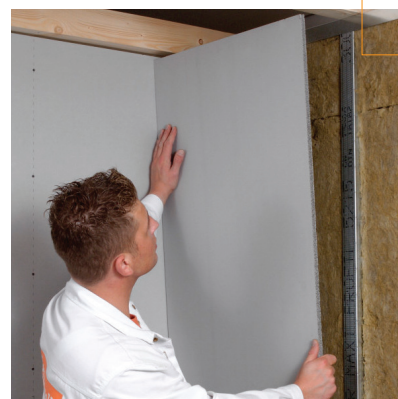
Powerpanel H 2 O can be fixed to steel or treated timber sub-structures.
