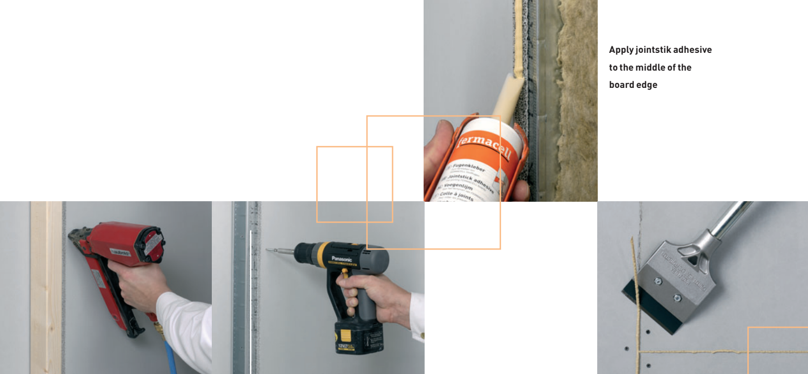
Staple or screw to the sub-structure
