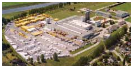
Calbe Factory, Germany
