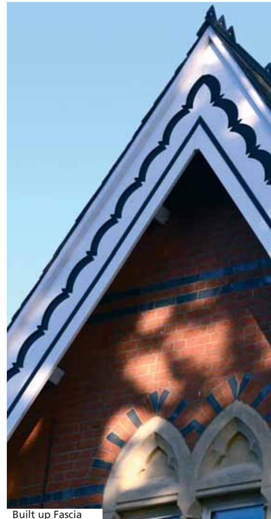
Built up Fascia
