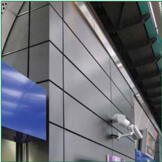
interior wall linings 4-5
