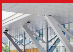
Fascia and soffits
