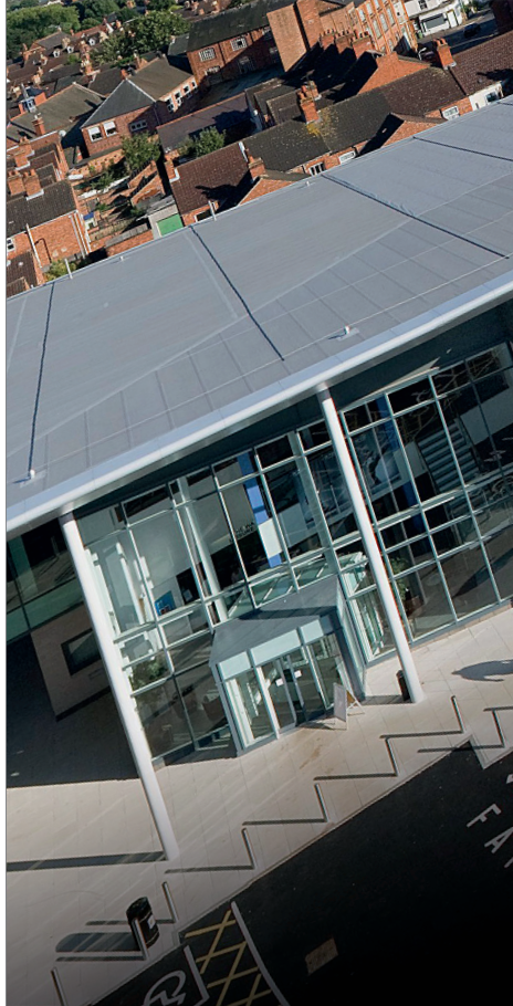
Cover image courtesy of IPS Group, North Yorkshire: Single ply membrane roof installation at the Waendel Leisure Centre, Wellingborough.
