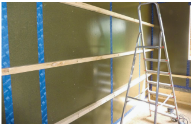
Durélis VapourBlock board sealed at joints with pro clima airtightness tapes as reliable internal airtightness and vapour control layer
