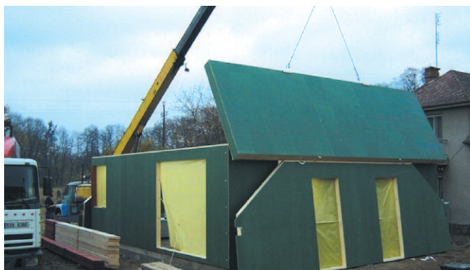
DURÉLIS POPULAIR board used as diffusion open racking board on site
