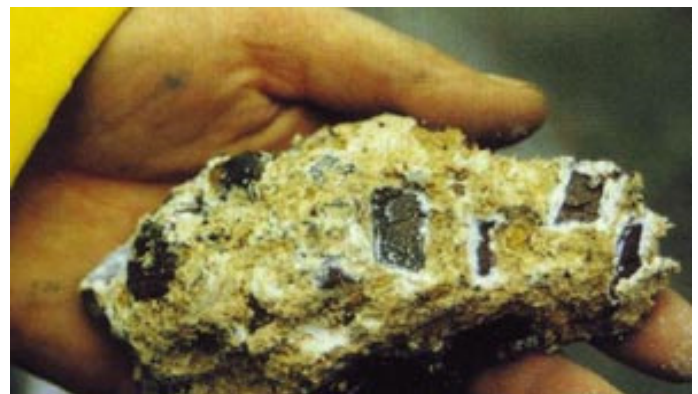
Concrete suffering Thaumasite degradation
