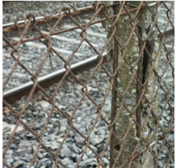
Chloride attack on concrete post
