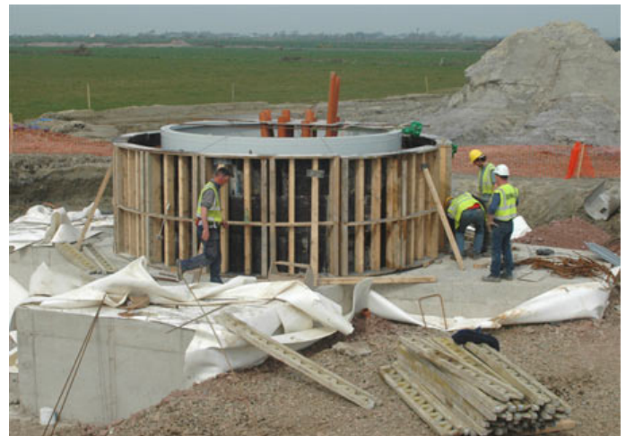
Multi-pile and reinforced concrete slab foundation near Kilmore Quay, Co. Wexford.
