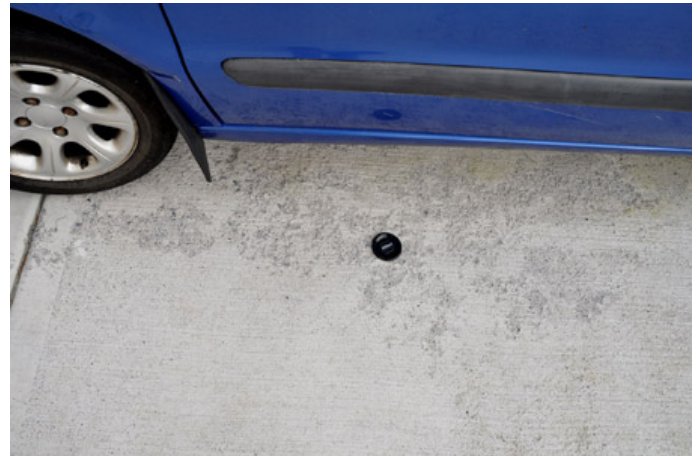
General disruption from freeze-thaw attack and the effect of de-icing agent melting from parked car
