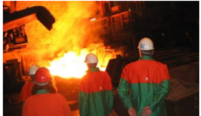
Molten slag en route from the base of the blastfurnace to the granulation vessel for cooling.
