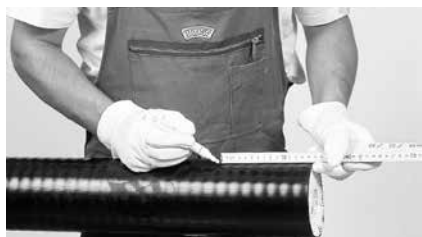
1 Mark the distance (x, y, z) + 1 cm from the end of the pipe.
