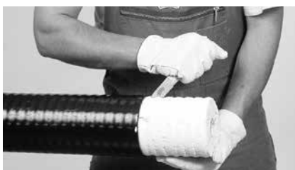
5 Cut back/remove the insulation along length (X, Y, Z). Note: Don't damage the carrier pipe!
