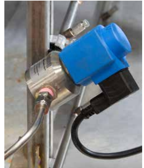
FIGURE 33-1: DRAIN VALVE AND DRAIN PIPING AT END OF MANIFOLD SECTION
