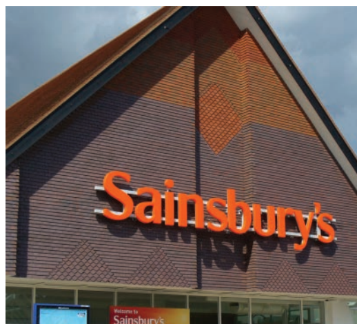
Below: The use of ornamental tiles and different colours for the vertical tiling produces a striking entrance to this supermarket.
