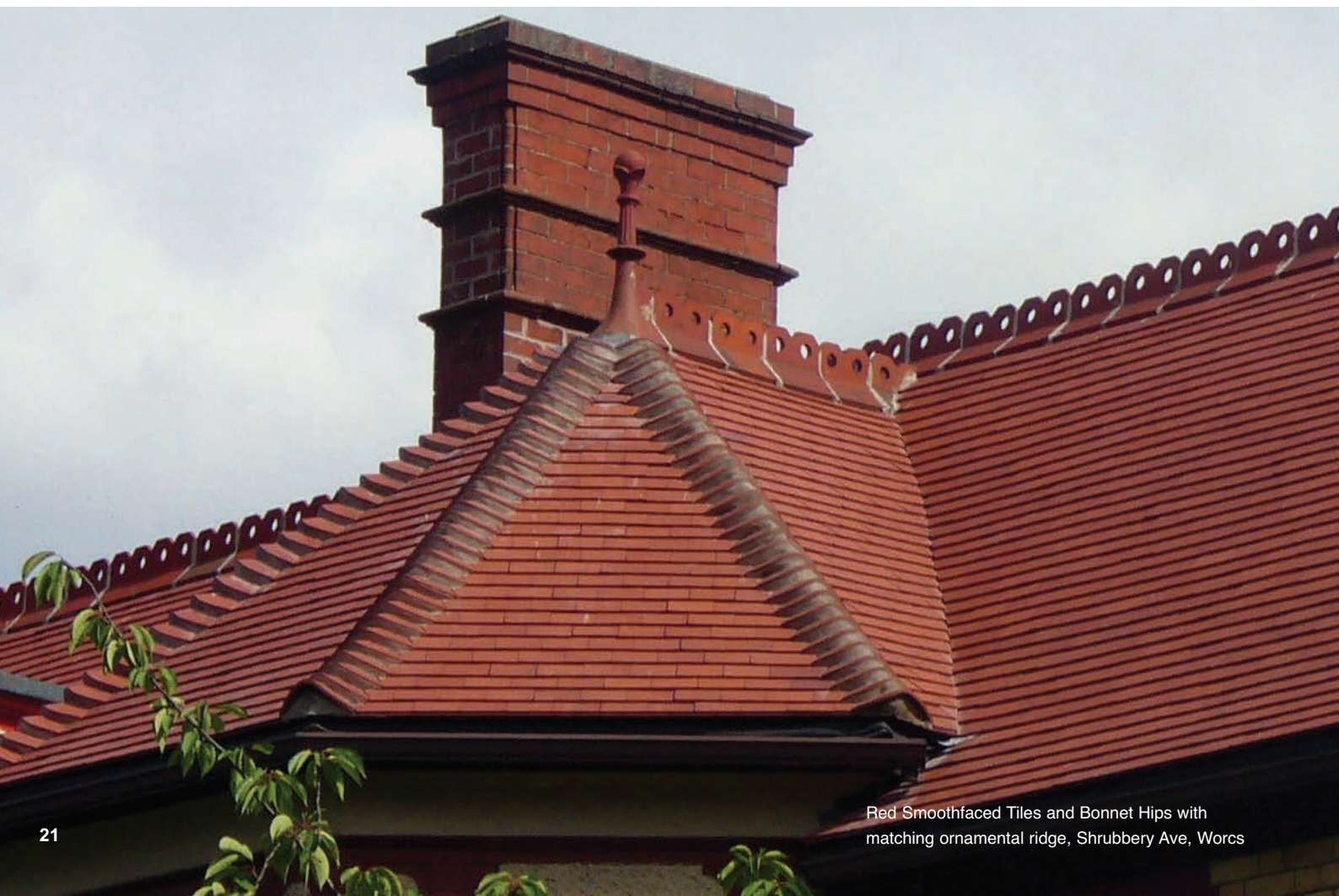
This Grade II listed Swiss style lodge, at Devonport Park, Plymouth, built in 1858, was refurbished with Red Dreadnought Ornamental Fishtail tiles.
