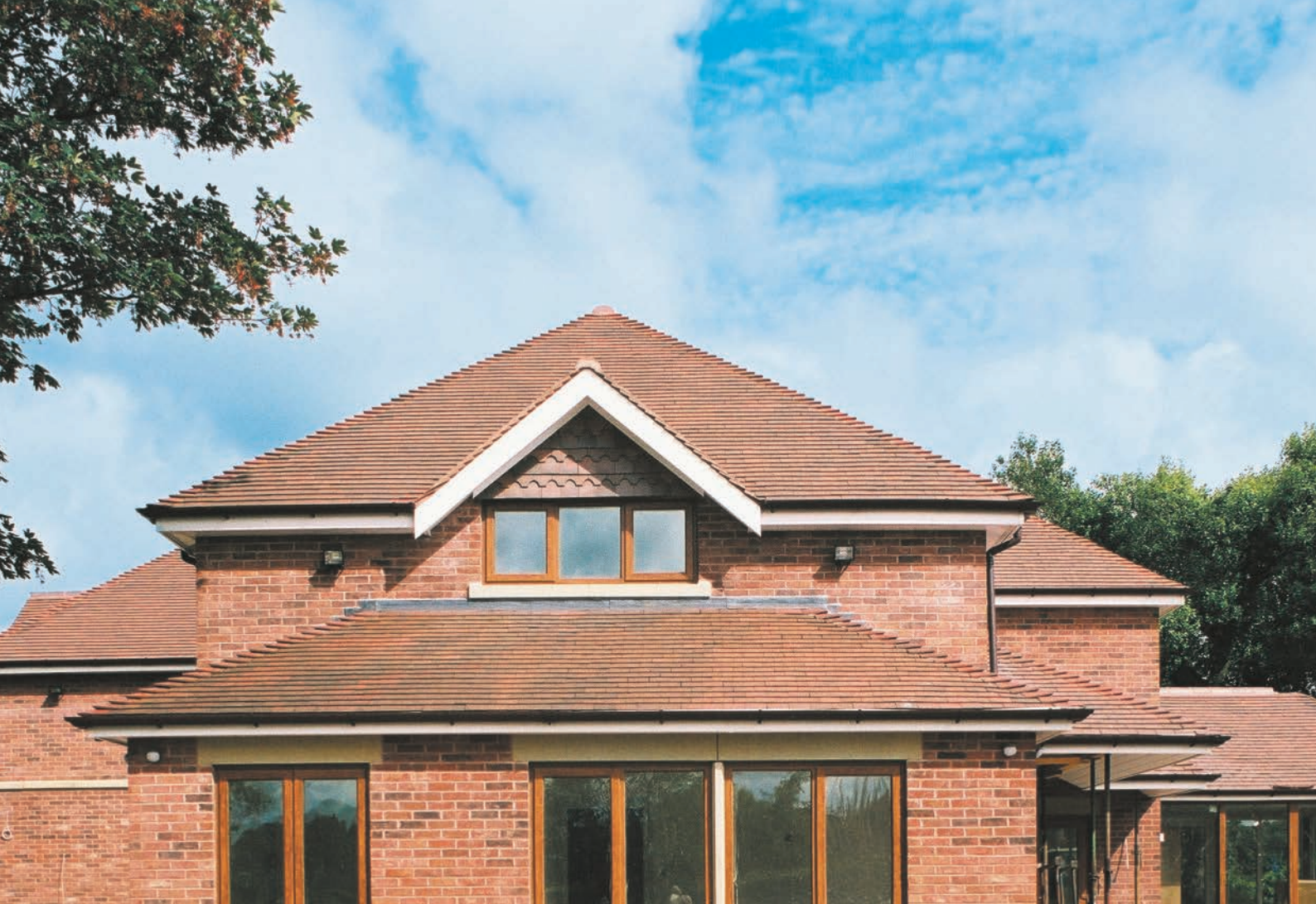
Above: The Brown Brindle Smoothfaced tiles on this private house in Lancashire, complement the lighter multi-coloured brickwork. The use of arris hips provides a neat finish to the hip lines on this stunning property.
