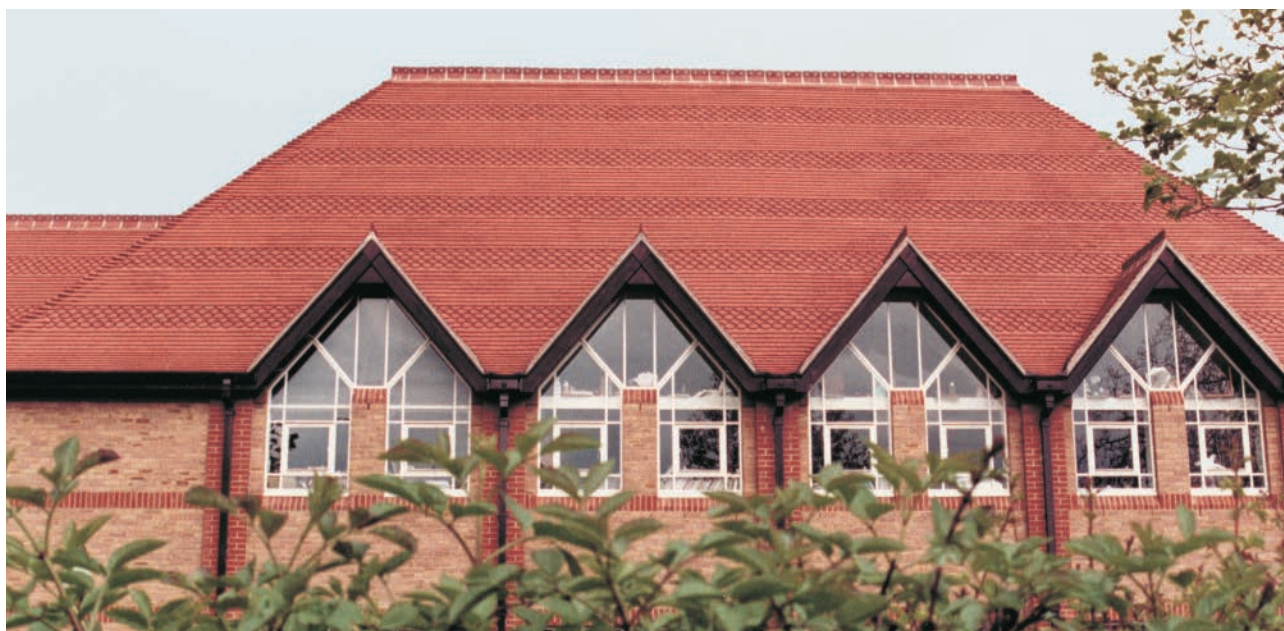
Below: Roding Valley High School, Loughton, Essex. This red sandfaced roof complements the buff and red brickwork. The large expanse of roof is broken up by the use of 5 bands of ornamental tiles, in alternating courses of club and fishtail tiles. The roof is topped with 2 hole ornamental ridges.
