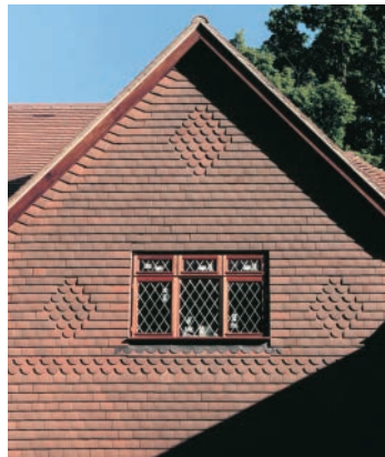
Left & Above: Brown Heather tiles have been used on the roof and vertical tiling on this house. Skillful and imaginative use of ornamental club tiles has enhanced the appearance of this building.
