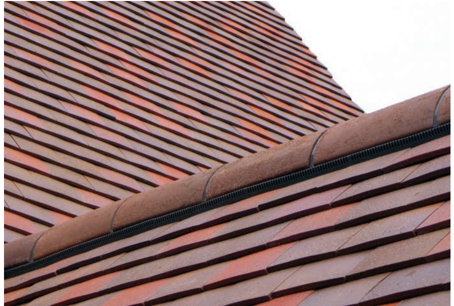
Above: A Dry Fix Ridge Vent on a private house in Dover
