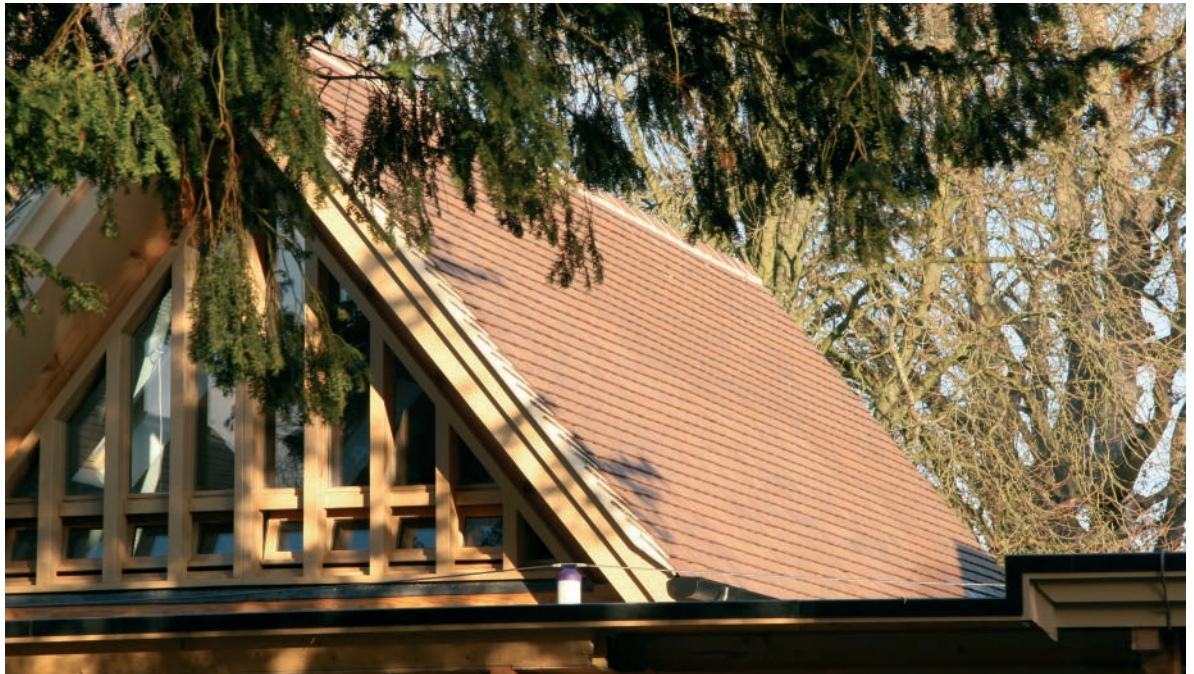
Right: Brown Heather Sandfaced tiles were chosen for the redevelopment of Micheldever Primary School.
