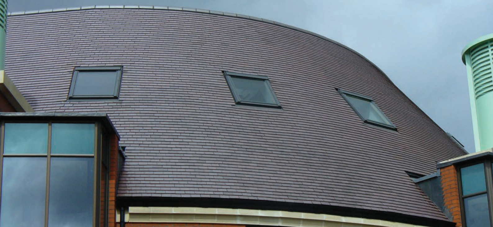
Above: This striking Library building in Swindon demonstrates the use of Staffordshire Blue tiles, a traditional product, in a contemporary design.
