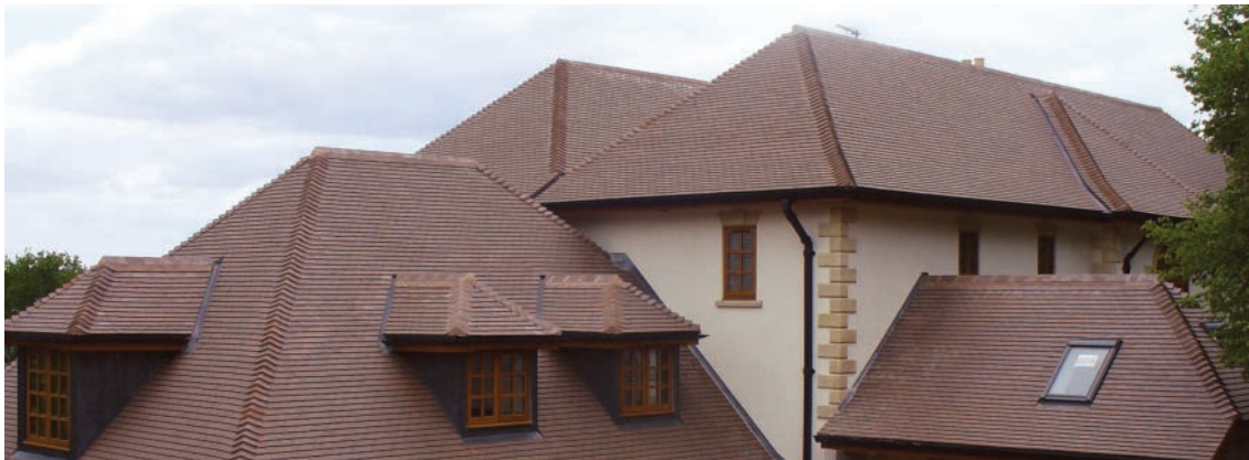
Left & Above: Brown Heather tiles have been used on the roof and vertical tiling on this house. Skillful and imaginative use of ornamental club tiles has enhanced the appearance of this building.
