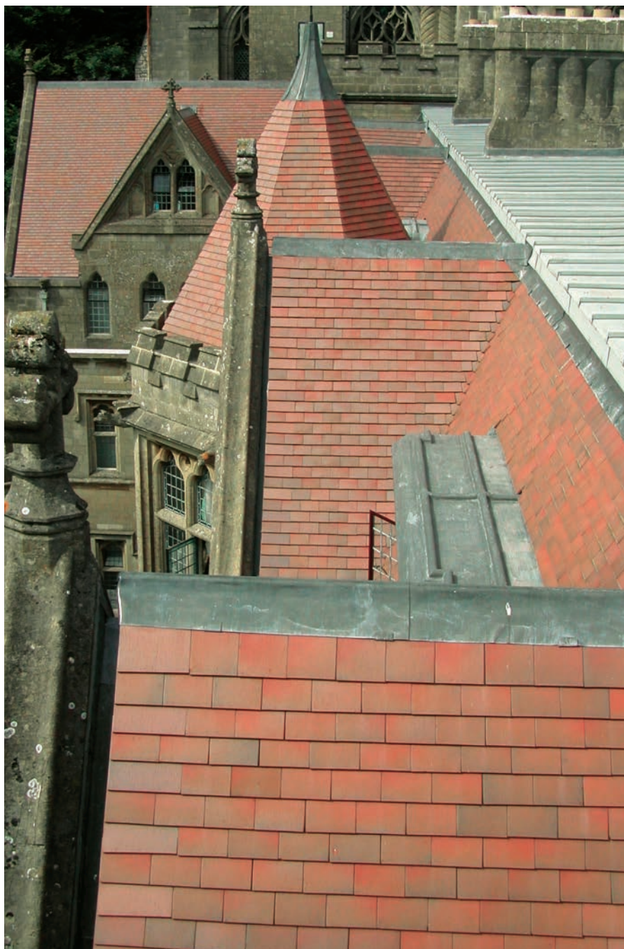
Above: Traditional single camber Country Brown Smoothfaced tiles were chosen for the re-roofing of Downside Abbey and this project was highly commended at 2008 Clay Roofing Awards.
