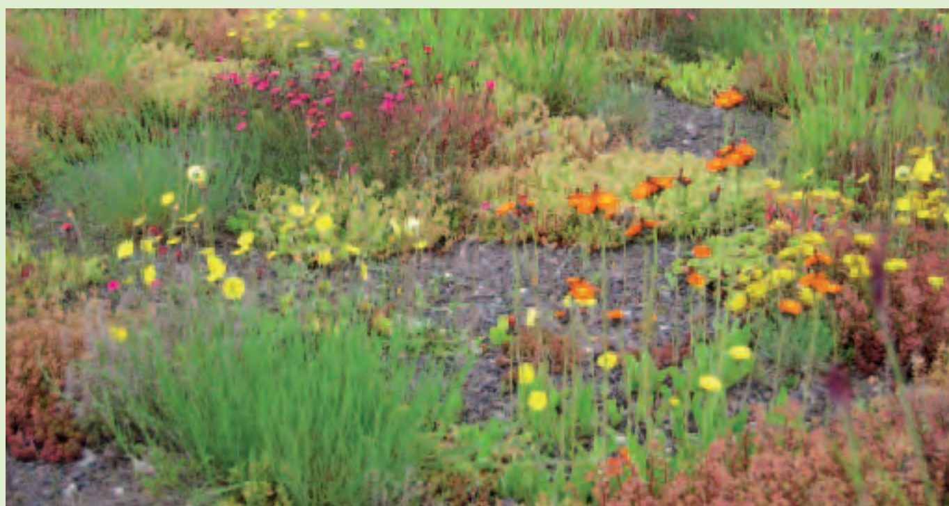
An extensive green roof
