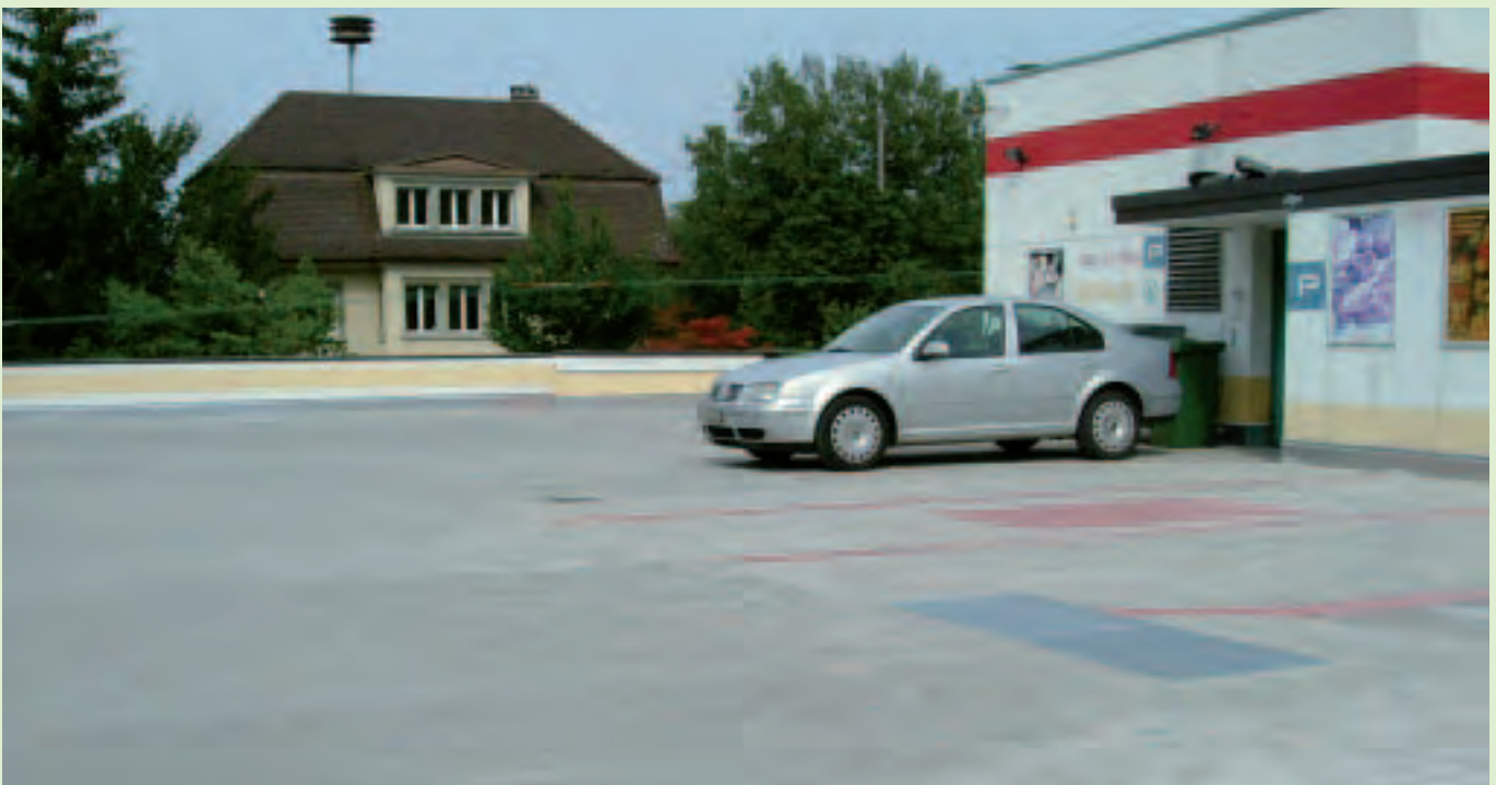
A drivable roof deck
