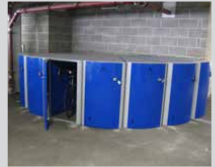
Seven Velo-Safe lockers were initially installed into the car park.
