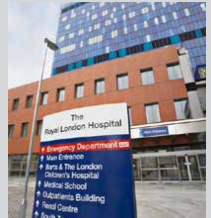
Cycle-Works were pleased to work with the NHS and Skanska on such a prestigious project.
