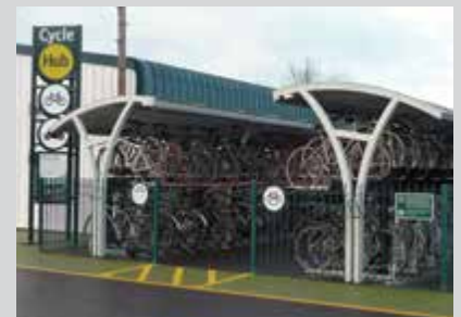
144 Josta 2-Tier Racks under the Cycle-Works Kennet Shelter.
