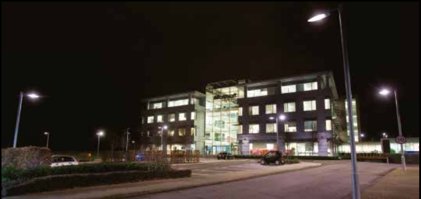
Microsoft Car Park - CU Phosco P567A Phosco LED Lanterns installed by others
