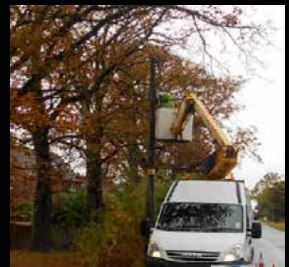
LED Replacement Lighting installed by CU INSTALLED
