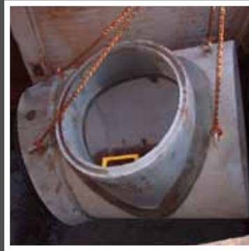
1200mm side entry complete with 10° bend
