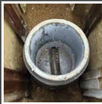
600mm sealed chamber base and chamber section
