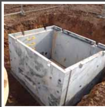
Flat pack complete with rebated chamber walls for access cover
