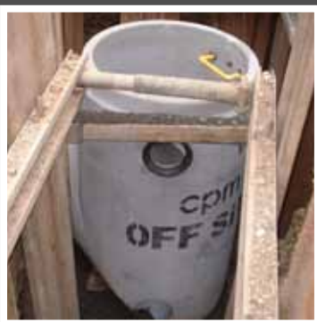
1200mm stop end bend complete with level inlet
