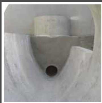
Ovoid channel and Internal back-drop junction in 2100mm chamber
