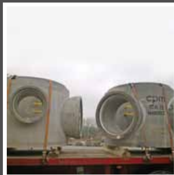
1800mm sealed manholes
