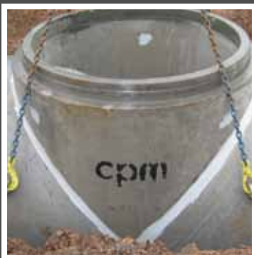
Sealed chamber installation
