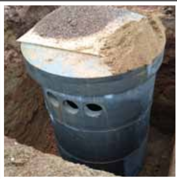
2100mm base chamber and section complete with pump pipework cut out in chamber wall
