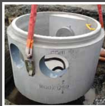
1800mm sealed chamber complete with Optimum Hydro-Brake®
