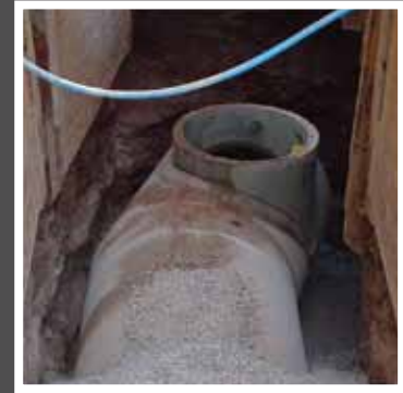
1500mm run entry complete with bend
