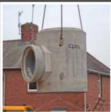
Single part 1800mm sealed manhole complete with pre-fitted 1200mm butt
