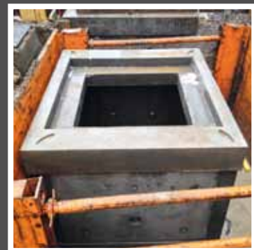
Flat pack chamber complete with rebated cover slab for access cover
