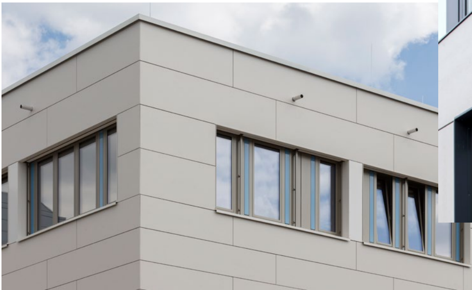
Erlangen Hospital (Germany)
