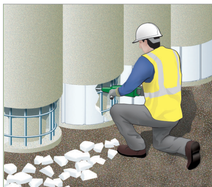
Excavated to basement level, Filcor is removed and pile reinforcement exposed.
