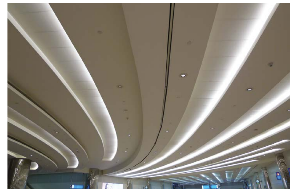
Suspended ceiling with SLAT™ (Self Levelling Access Trim) the unique patented Coopers' system
