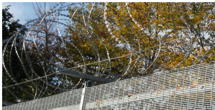
RAZOR WIRE INSTALLATION (ABOVE)
