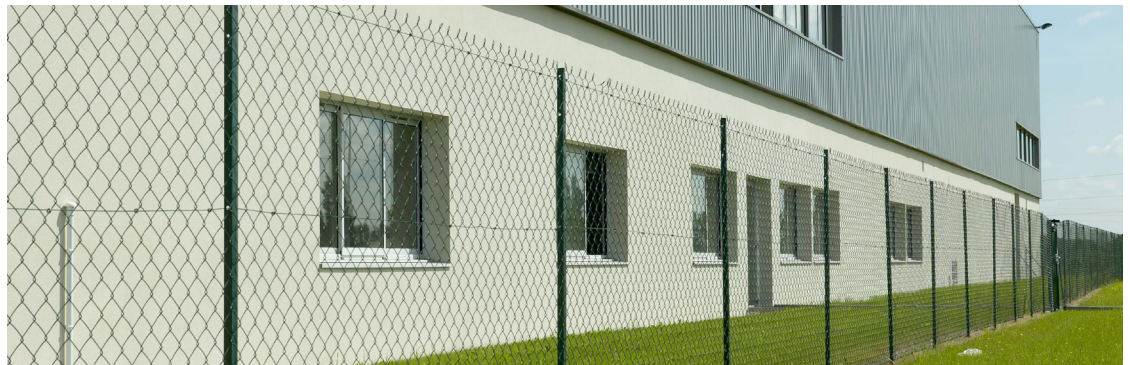
CHAINLINK INSTALLATION (ABOVE)
