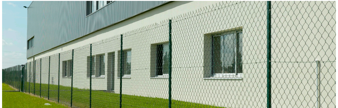
CHAINLINK INSTALLATION (ABOVE)
