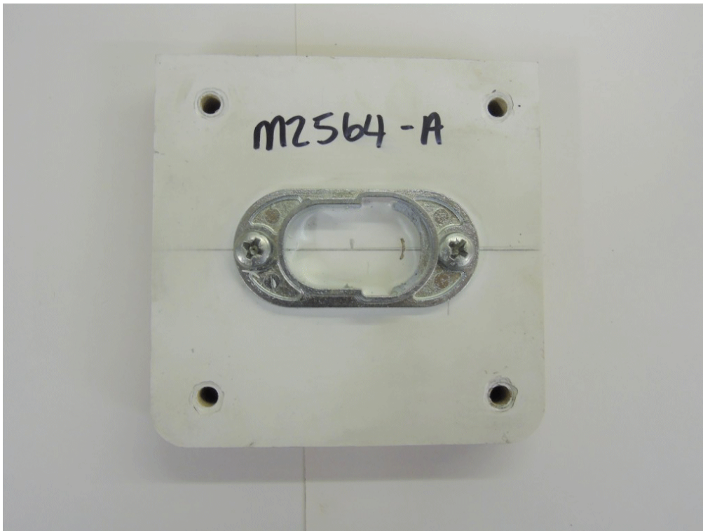
Photograph 2 A view showing the general condition of the fixing after a vertical shear test on a type 1 - metal fixing.
