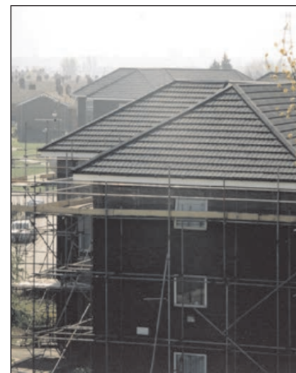
0.45mm Ultratile on a 3000m 2 Flat to Pitch project in Walsall.
