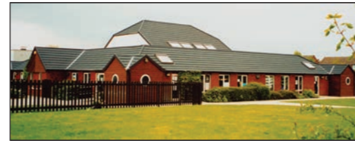
This school project used the 0.9mm thick Slate 2000 because of the high vandalism.
