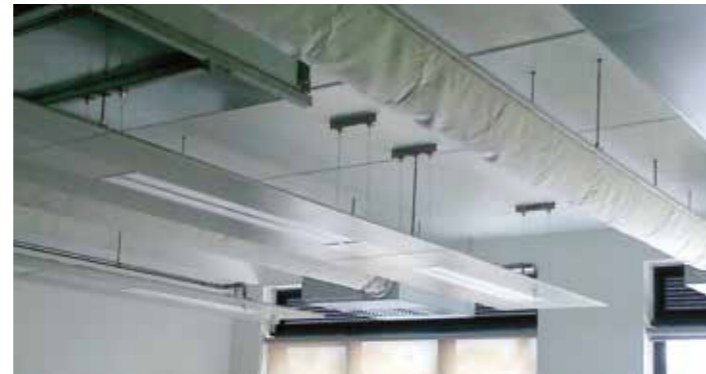
Figure 1: Fabric sock ducting arrangement
