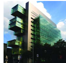
Civil Justice Courts, Manchester
