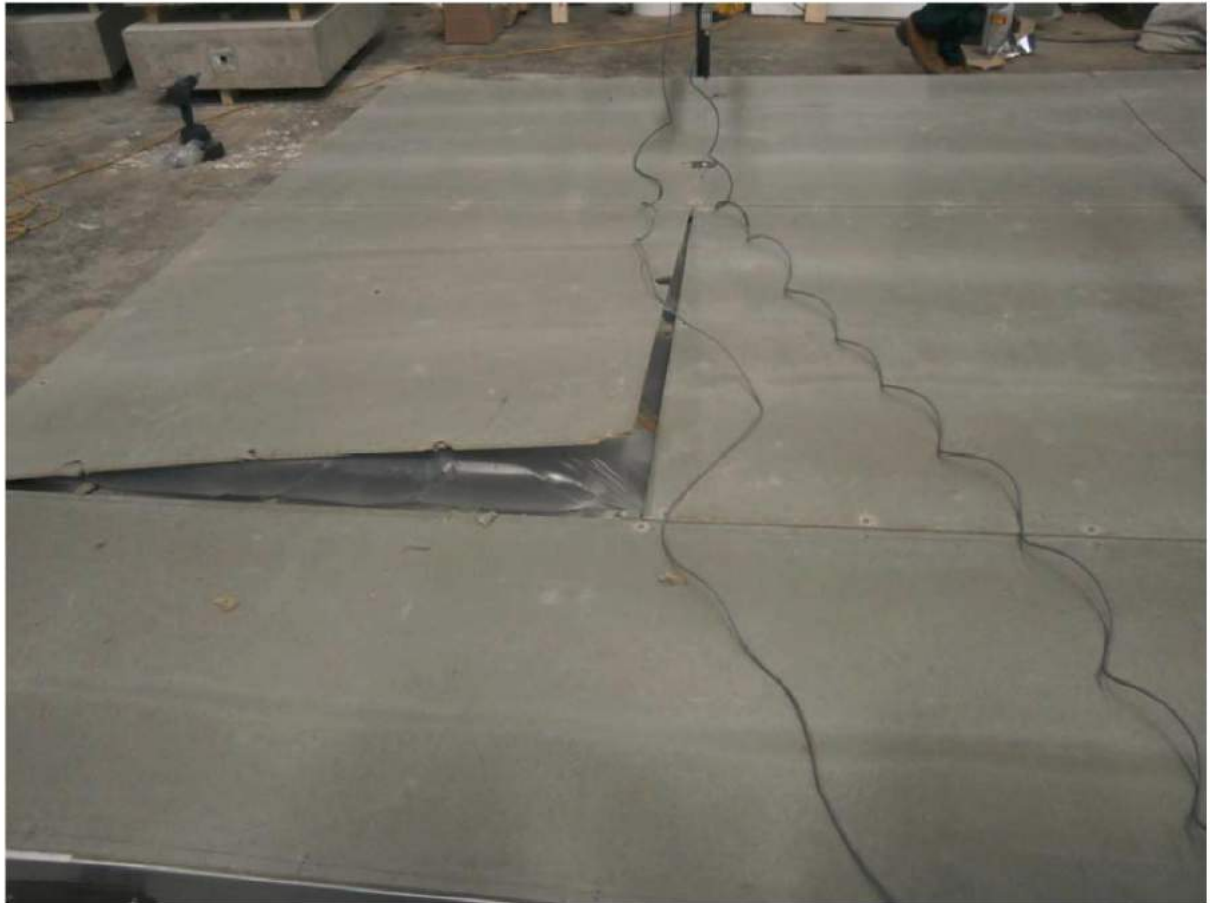
Plate 2 – Showing Failure of Half Board Pulling Away from Fixings
