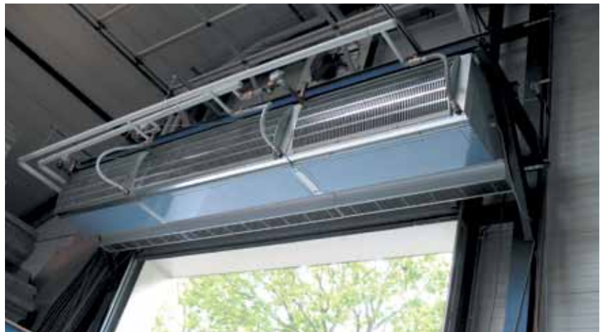
Model IndAC combines well with overhead door systems.
