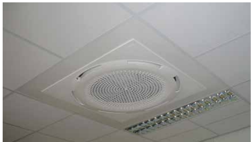
Using an adaptor plate the CC 90 is tailored to the existing ceiling system.
