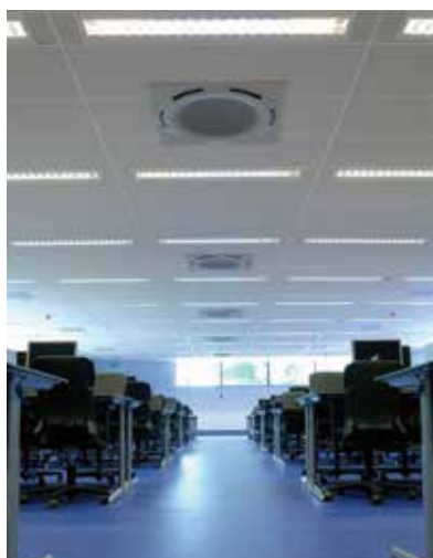
Biddle cassette units (CC 90) are in use in the computer rooms of this university.
