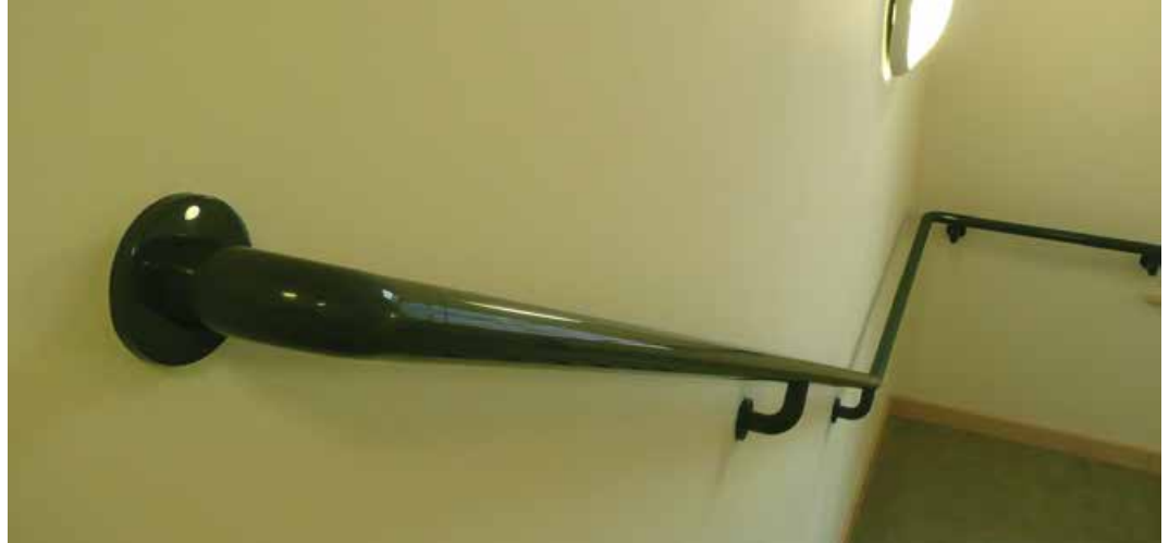
HANDRAILS (Section L30 clause 580 of NBS)
