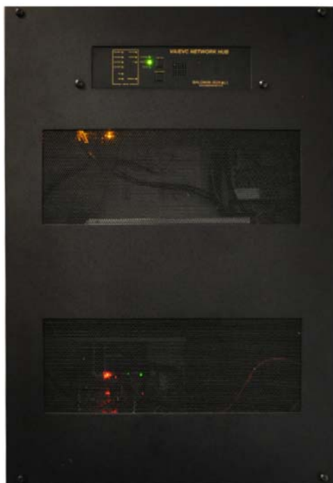
Figure 1.3 — Typical EVC Network Hub
