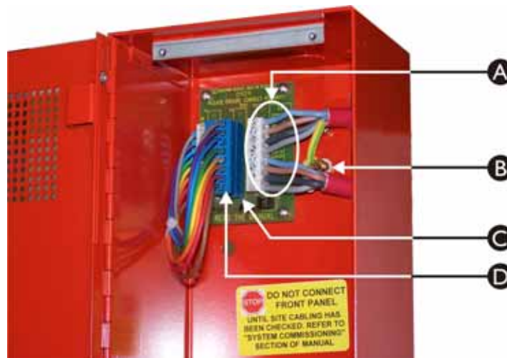
Figure 3.8 — BVOCC Termination Board and Typical Site Wiring
