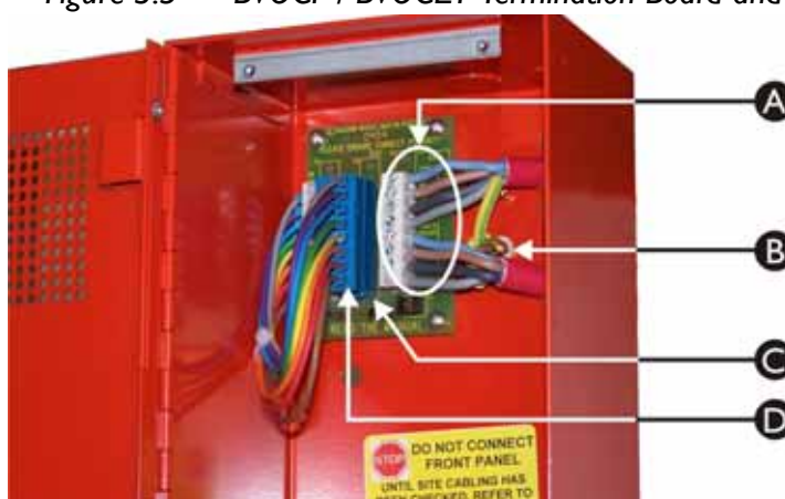
Figure 3.5 — BVOCF / BVOCET Termination Board and Site Wiring
