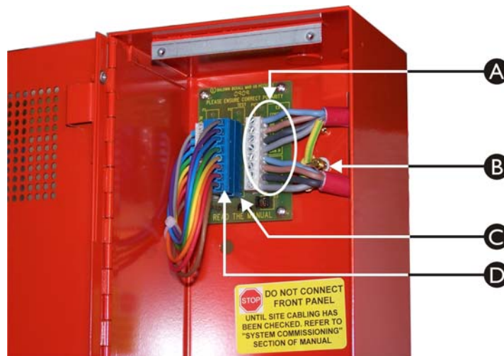
Figure 3.8 — BVOCC Termination Board and Typical Site Wiring
