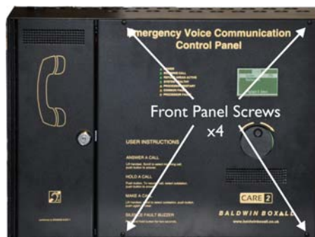
Figure 2.11 — Remove 4 x Front Panel Screws
