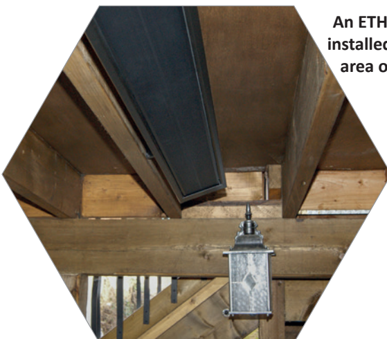
ETH Terrace heaters installed indoors in a football clubhouse in Norfolk
