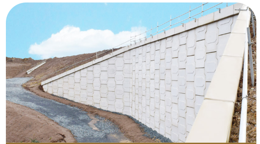
RETAINED EARTH WALL
