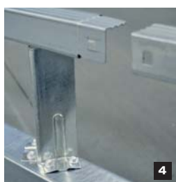
4/5. Once the Ashgrid bar is in place, the next bar may then be connected to it, by locating the open end onto the 'Safe-Loc' spigot and pushing firmly until the tab clicks into position. This bar may then be snapped onto the brackets as before
