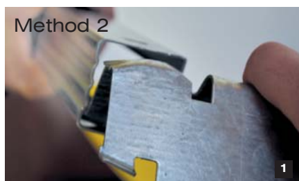
1. Position the Ashgrid ABV Bracket at the open end of the AG40 Bar
