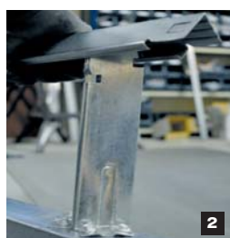
2. After laying the insulation (omitted from the photograph), position the AG40 bar onto the brackets, with the 2 'wings' located in the short downstand of the AG40 bar
