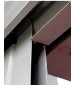
Guide & bottom rail interface
