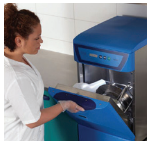
The sluice room
