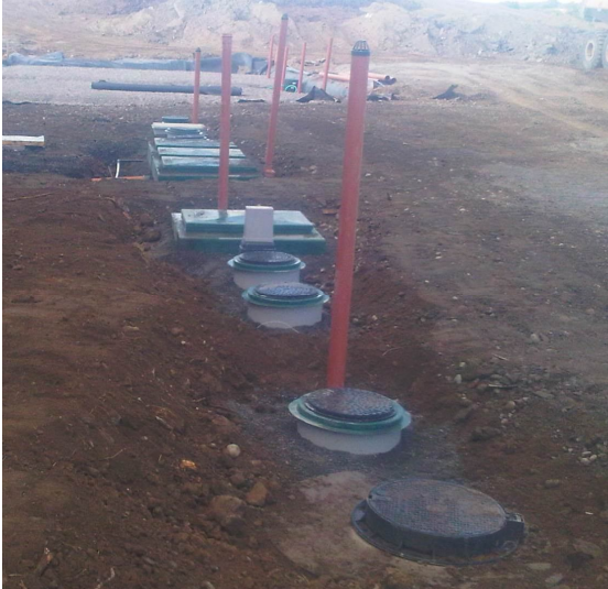
Figure 6 – Example of Units Vent Pipework
