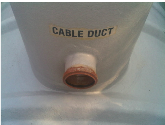
Figure 7 - Socket for 110mm Ducting
