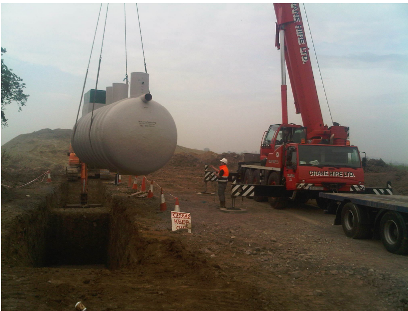
Figure 2 – Large Cylindrical Tank being installed
