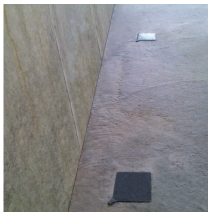
Void formers shown at Slab-to-Wall joint
