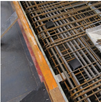
Reinforcement being located around ESDQ-L20 Sleeves
