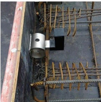
HLDQ-L30 Sleeve nailed to formwork
