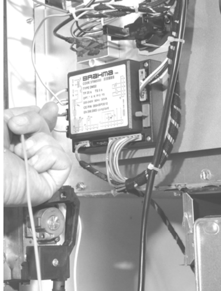
Figure 22 Disconnect wire of the ignition electrode at the burner controller
