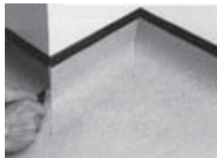
4. Cut in the front external mitre.
