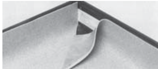
4. This completes the first part of the mitre.
