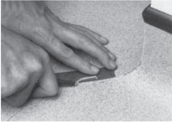
1. Groove the floor and bottom section. The top section of the mitre forms a natural 'Vee' and does not need grooving.
