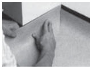
3. Take a separate piece of flooring roughly cut to size, apply adhesive, position and cut to fit the back internal mitre.
