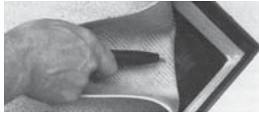
2. Make a cut from the base out to the top of the flooring in line with the mitre.
