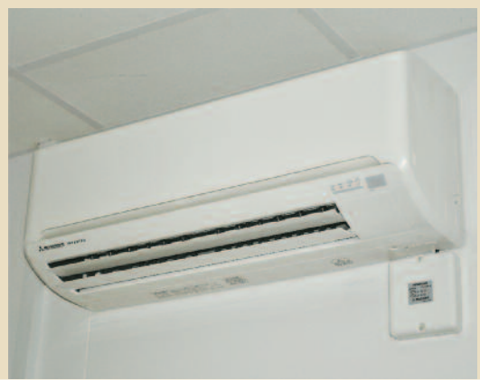
► Wall mounted airsource heat pump heating system (split system) Provides the most cost effective heating system available.
