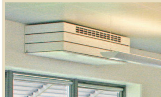
► Heat recovery system Provides sufficient ventilation to your working space without losing heat to the atmosphere thus minimising carbon emissions and saving you money.
