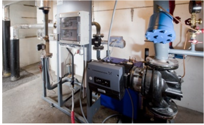
The inner network is connected to the exterior loop via a Maxi station.
