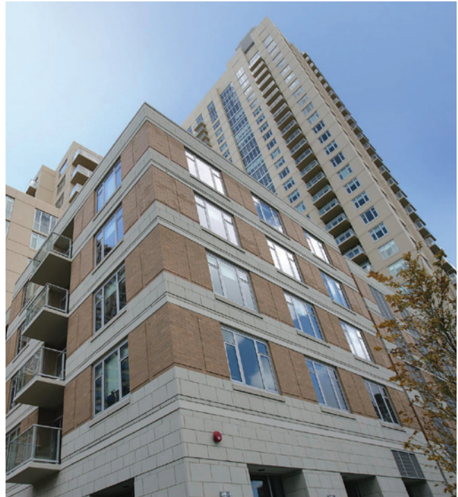
The Admiral at the Lake, Chicago, Illinois, USA Architect: Perkins + Will, Dallas, Texas, USA Window Installer: Softer Lite Window Company, Chicago, Illinois, USA Traco TR-700 Window Wall with Traco TR-710 – 4-5/8" Offset Casement Thermal Aluminum Windows (Outswing) Traco TR-750 – 4-5/8" Offset Projected Thermal Aluminum Windows (Project Out) Traco TR-780 – 4-5/8" Offset Depth Fixed Thermal Aluminum Windows
